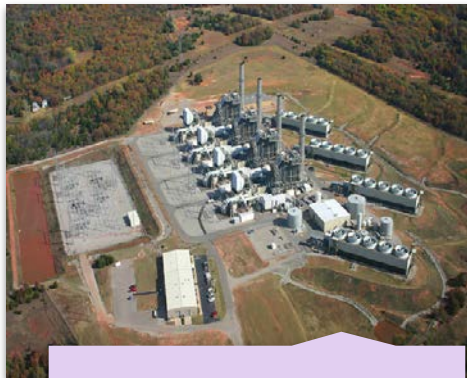
443 MW Combined Cycle Gas Redbud Power Plant
