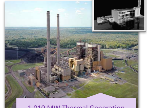
1,010 MW Thermal Generation Grand River Energy Center 495 MW Combined Cycle Gas currently under construction
