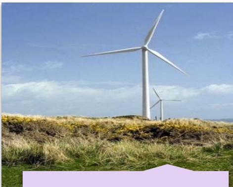
247 MW Wind Generation Combined across three projects
