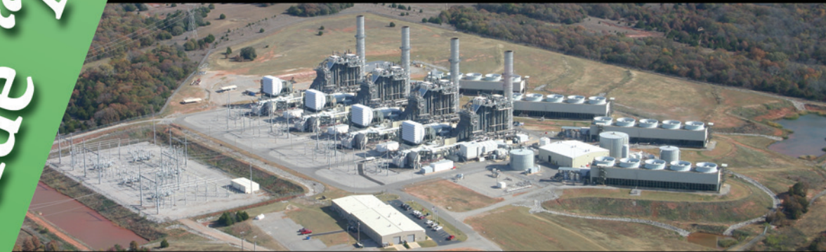
Redbud Plant, Luther, OK
