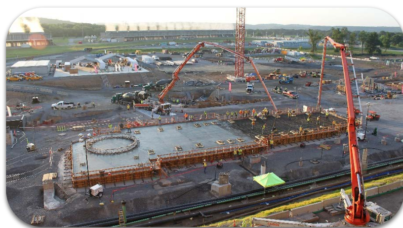
A concrete pour at Grand River Energy Center created the foundation for the new Heat Recovery Steam Generator as part of the ongoing Unit 3 construction.
