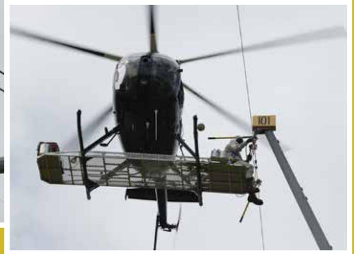
GRDA contractor Haverfield Aviation, Inc. performed helicopter operations during September along a high voltage power line running between GRDA's Grand River Energy Center (formerly Coal Fired Complex), and the Tonnece Substation near the Arkansas state line. The work consists of the helicopter hovering above each transmission structure as a lineman removes old insulating components from each structure. The line remains energized while the lineman performs the work.
