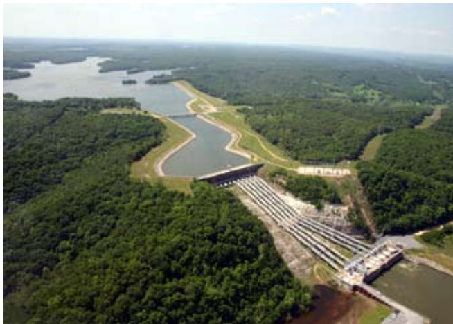
On the job... Chancellor oversees the maintenance operations of the GRDA Salina Pumped Storage Project.
