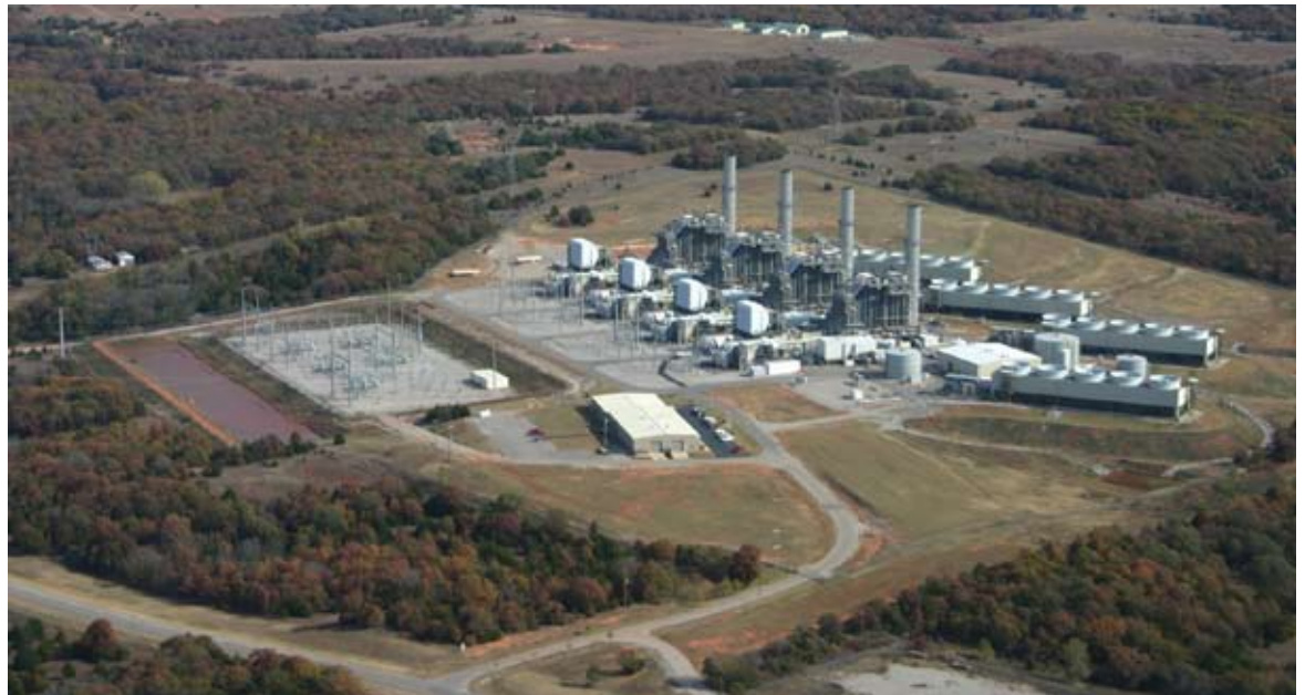
An aerial view of the Redbud Power Plant (Luther, Okla.).
