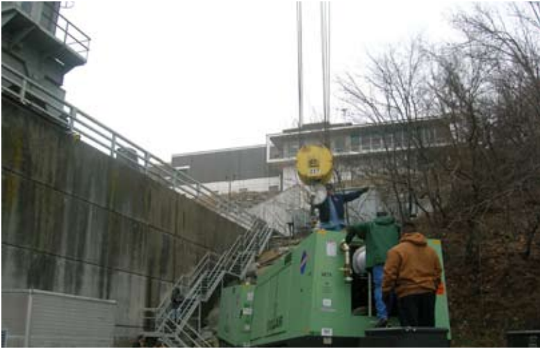
GRDA crews and contractors unload air compressors to be used for forced air testing procedures at GRDA's Robert S. Kerr Dam.
