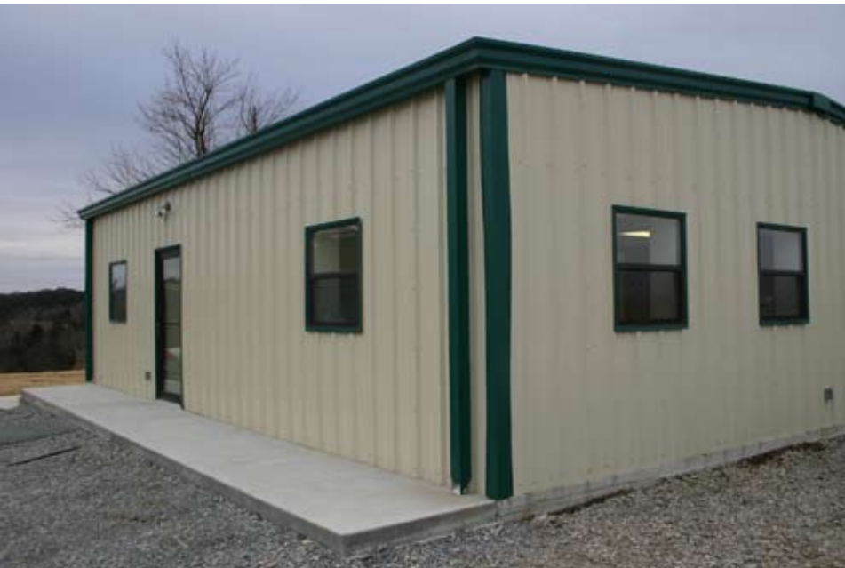
This building, home to GRDA’s Cushing Line Crew, was constructed by the PMD.
