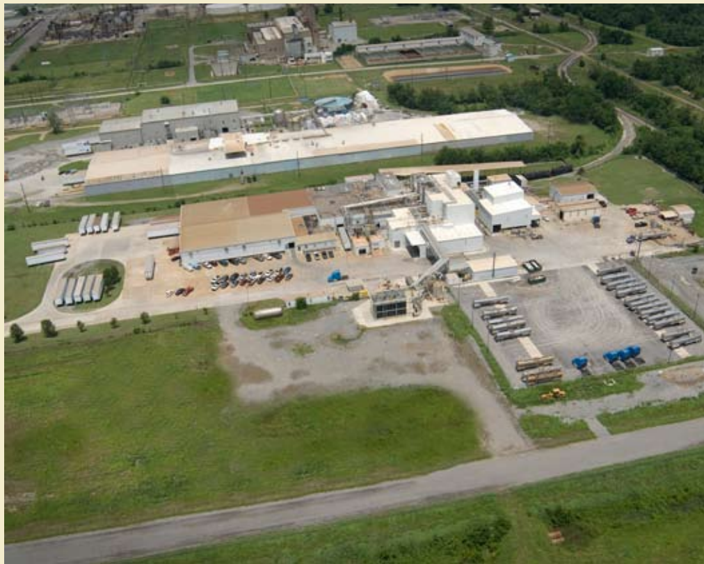
Interplastic, a MidAmerica Industrial Park facility.
