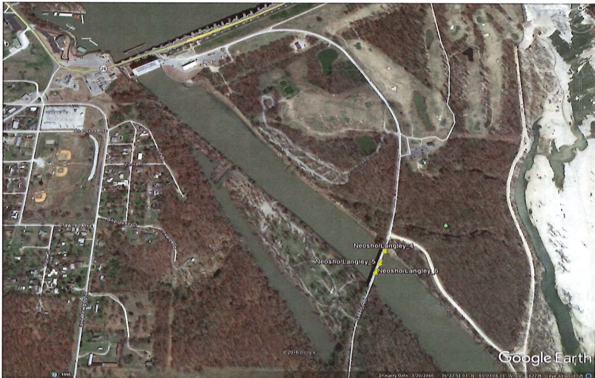
Figure 1 Testing Sites for Pensacola Dam
