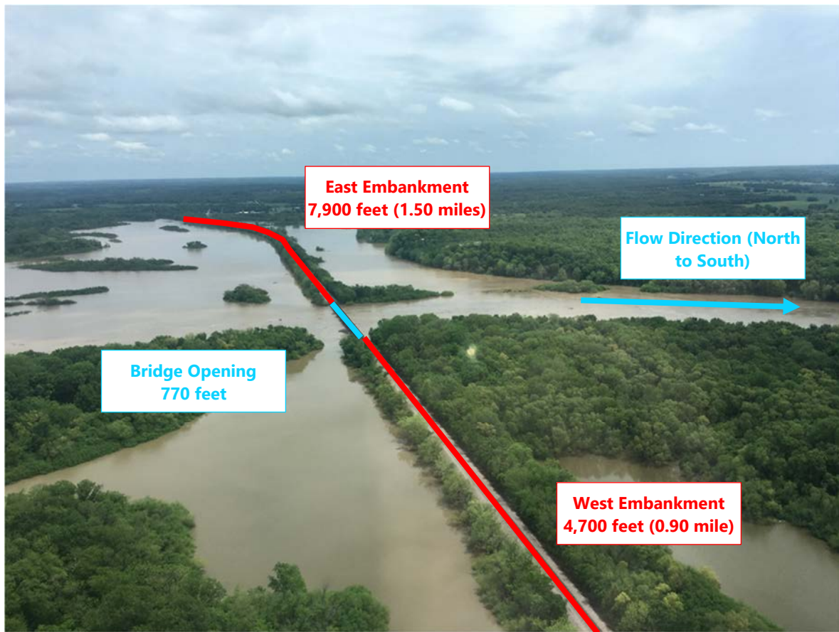
Figure 71 Burlington Northern Railroad Bridge and Embankment near Twin Bridges Photograph Looking East
