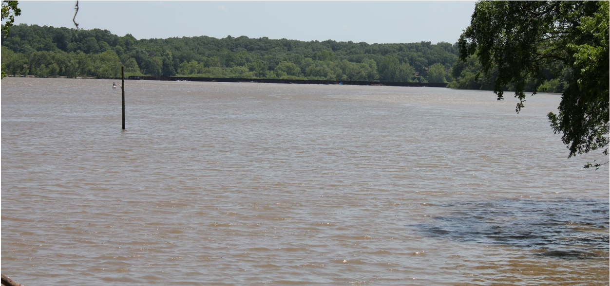
Figure 130 Burlington Northern Railroad Bridge and Embankment Viewed from Twin Bridges Boat Launch in May 2019
