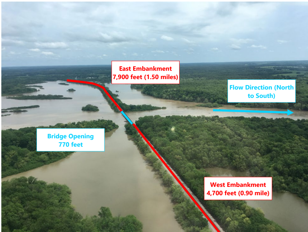
Figure 71 Burlington Northern Railroad Bridge and Embankment near Twin Bridges Photograph Looking East
