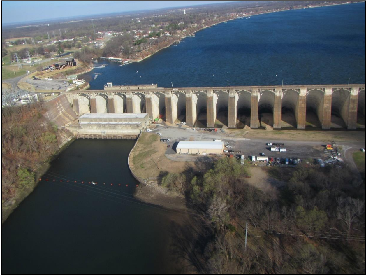
Figure 3.10.1-1 Pensacola Dam, Powerhouse and Tailrace Looking Upstream
