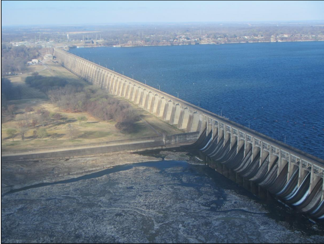
Figure 3.10.1-2 Pensacola Dam Looking West
