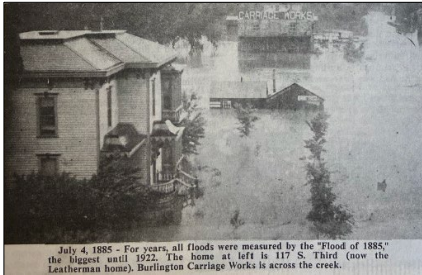
Figure 1. Neosho River flood, Burlington, Coffey County, Kansas, July 4, 1885.
