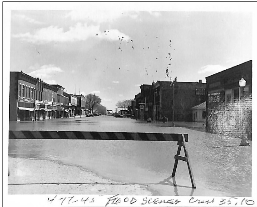
Figure 34. Neosho River flood, Burlington, Coffey County, Kansas, April 17, 1945.
