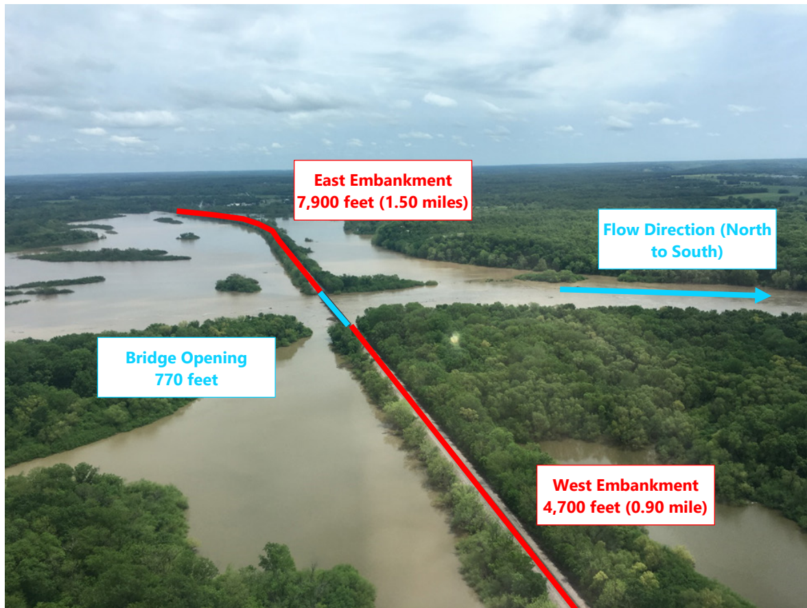
Figure 69 Burlington Northern Railroad Bridge and Embankment near Twin Bridges Photograph Looking East
