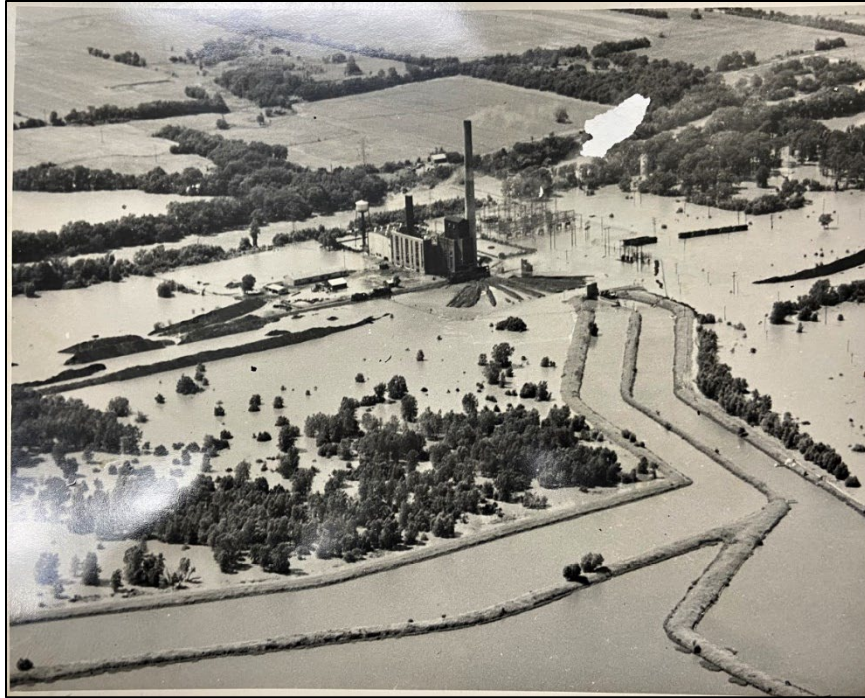
Figure 38. Neosho River flood, Kansas Gas & Electric plant, east of Parsons, Labette County, Kansas, July 25, 1948.
