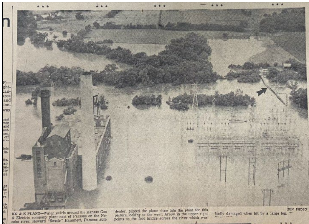
Figure 43. Neosho River flood, Kansas Gas & Electric plant east of Parsons, Labette County, Kansas, July 14, 1951.
