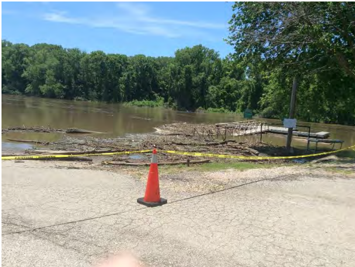
6. Twin Bridges State Park (lower) – May 30, 2020; view west. Site flooded. High water level recorded at 748.29 feet.
