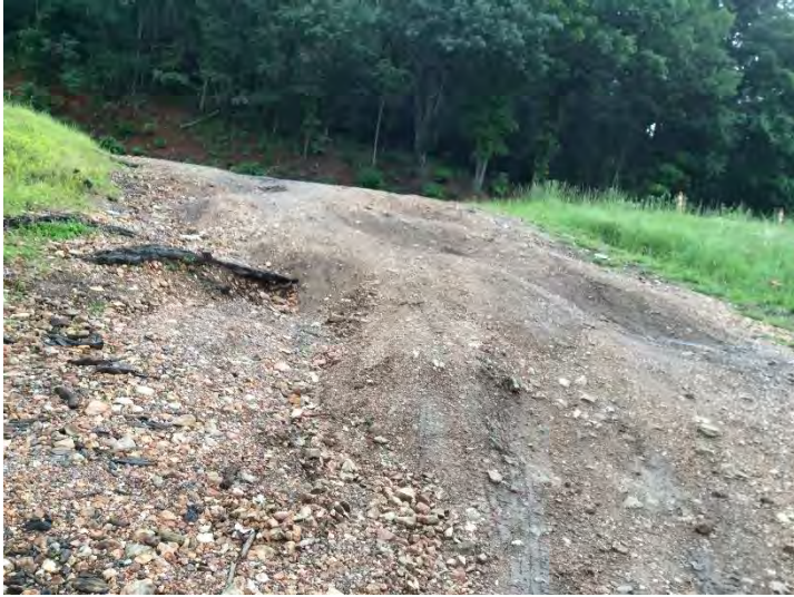
1. Council Cove – May 22, 2020. View east of boat ramp access. Parking area above and to left.
