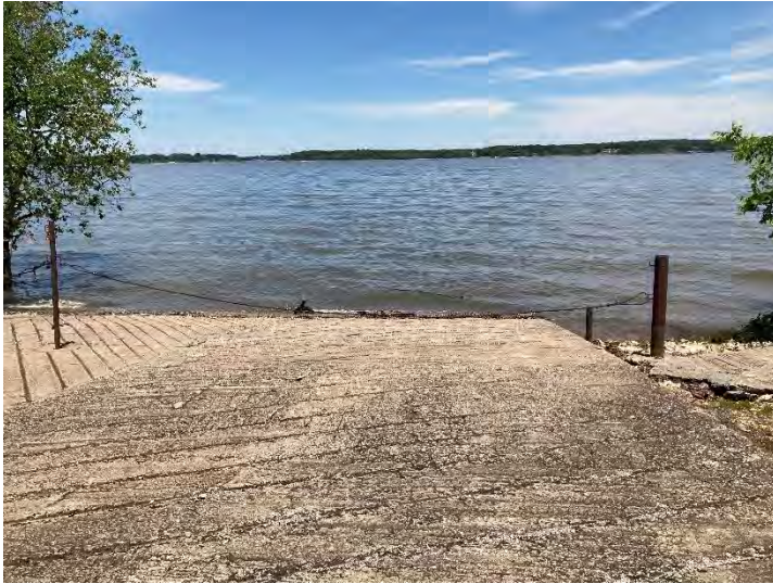
28. Cherokee State Park at Disney – May 30, 2020; view north. High water level recorded at 748.29 feet. Ramp closed.
