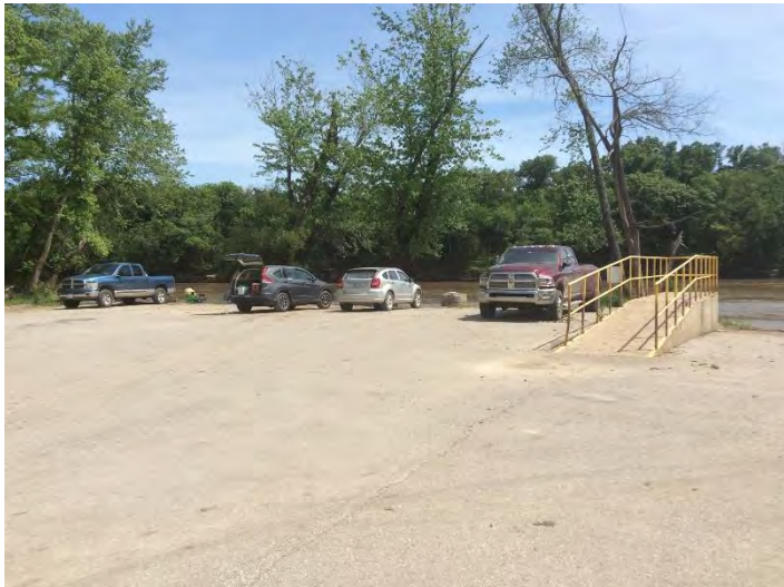
3. Connors Bridge – May 23, 2020. View west of parking area and ramp.
