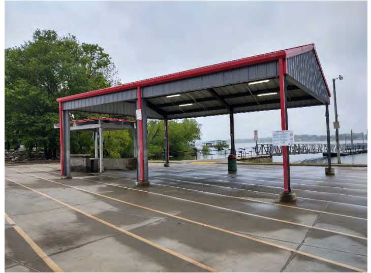
2. Wolf Creek – May 12, 2020. View north of mini pavilion.
