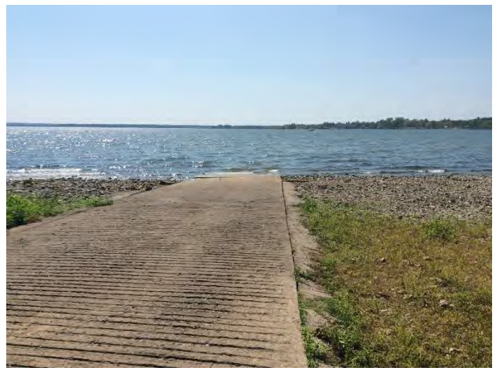
43. Bernice State Park – September 26, 2020; view southwest of south ramp. Low water level recorded at 742.2 feet.
