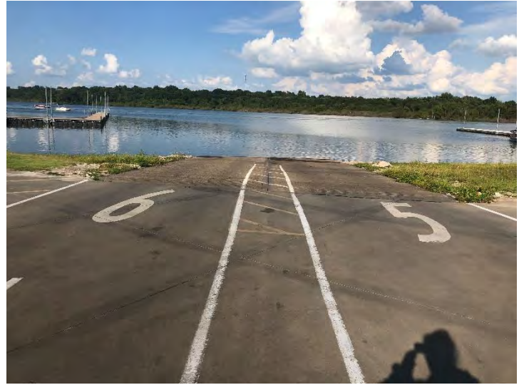
10. Wolf Creek – September 4, 2020. View northeast of boat ramps.
