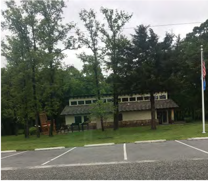
5. Twin Bridges State Park, Upper – May 2020. Administrative offices and Nature Center
