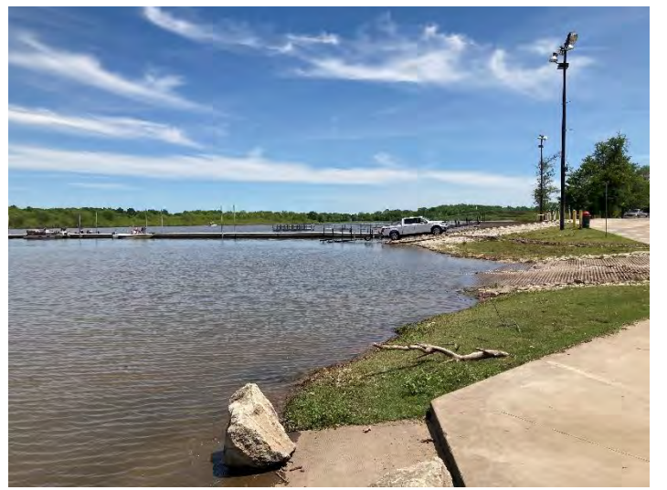
4. Wolf Creek – May 23, 2020. View southeast of boat ramps.
