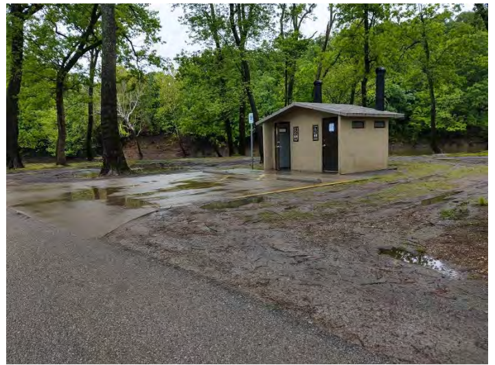
2. Cherokee State Park, Riverside (west) – May 12, 2020. View south from parking area of restroom.
