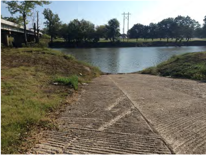
5. Riverview Park Site B – September 26, 2020; view east. Low water level recorded at 742.2 feet. (no high water mark photo from May available)
