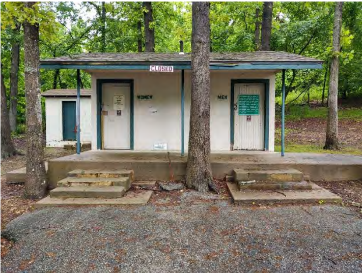
3. Honey Creek State Park – May 12, 2020. View south of restroom facility in boat trailer parking/camping area.
