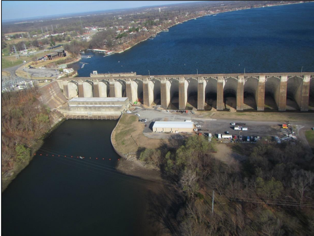
Figure 3.10.1-1 Pensacola Dam, Powerhouse and Tailrace Looking Upstream
