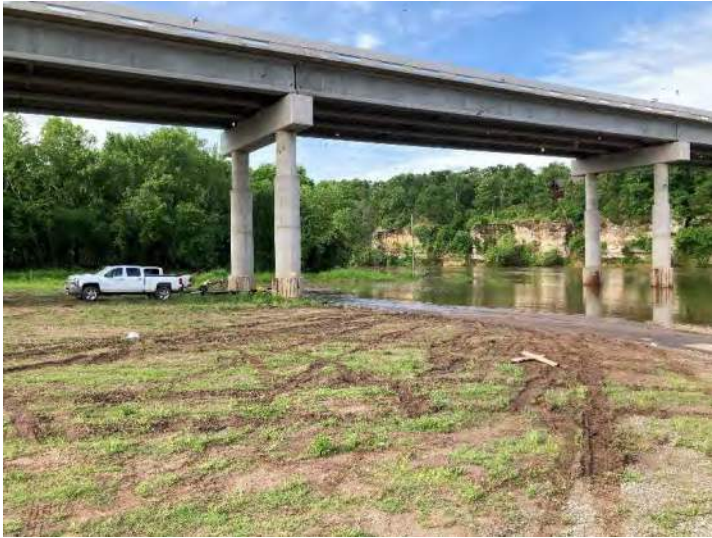
1. Spring River – May 17, 2020. View SW from parking area.
