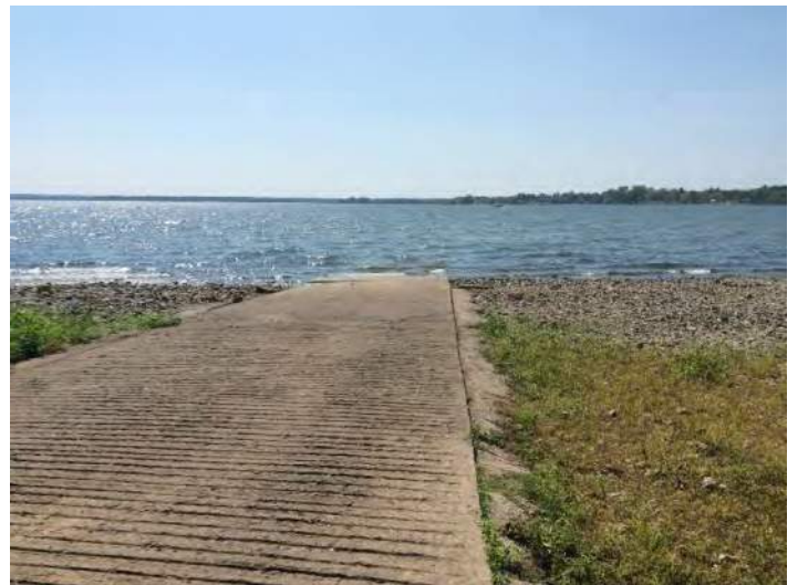
43. Bernice State Park – September 26, 2020; view southwest of south ramp. Low water level recorded at 742.2 feet.
