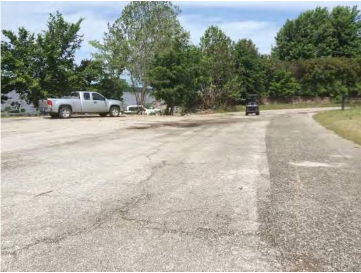
1. Monkey Island – May 23, 2020. View west of parking area toward ramp.
