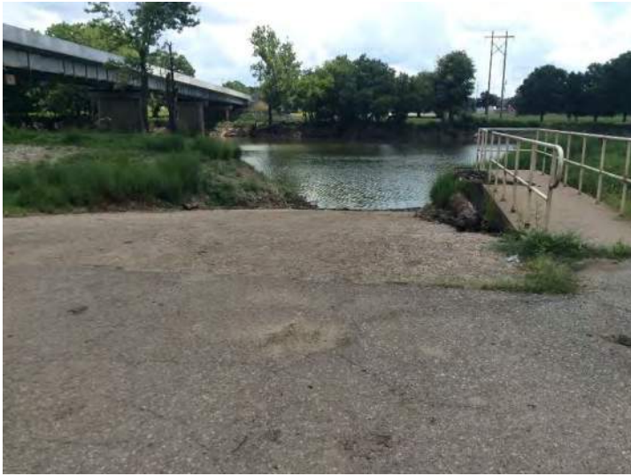
1. Riverview Park Site B – July 5, 2020. View east of boat ramp from parking area.
