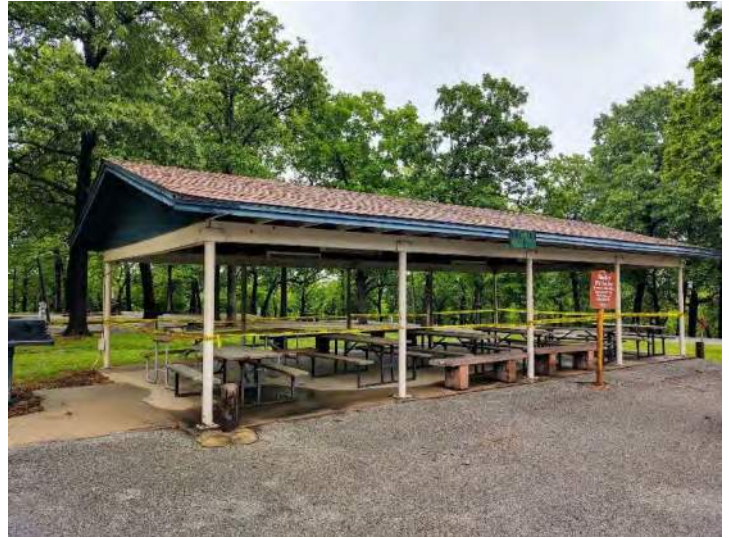
6. Honey Creek State Park – May 12, 2020. View north of pavilion near shower facility and camp sites.
