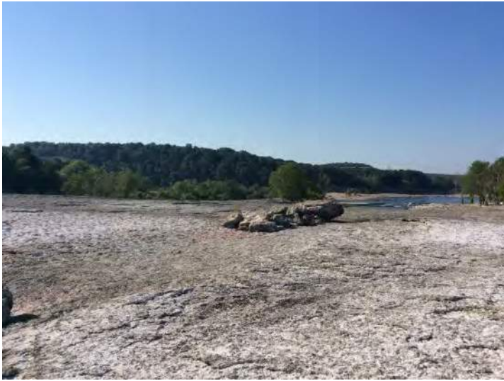
1. Channel Site – June 18, 2020. View southeast of area below Pensacola dam spillway.
