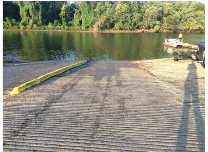
7. Twin Bridges State Park (lower) – September 26, 2020; view west. Low water level recorded at 742.2 feet.
