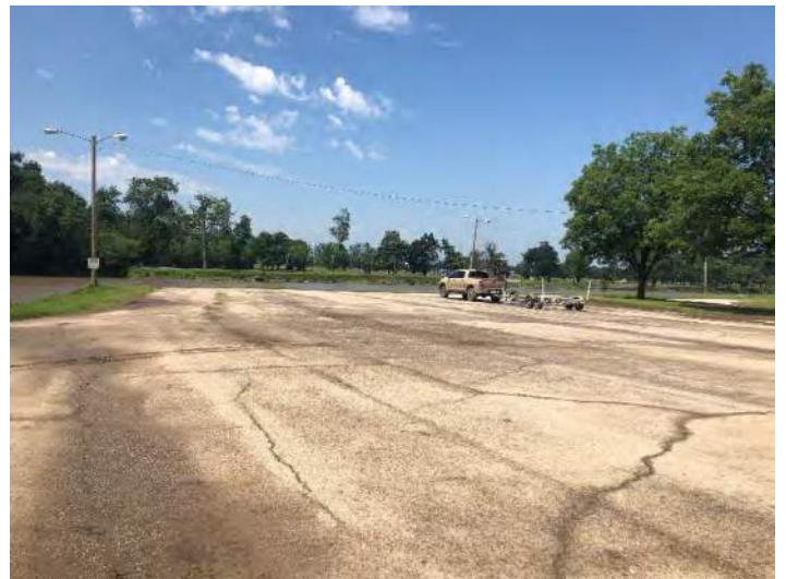
4. Riverview Park Site A – August 8, 2020. View west from parking area near boat ramp.
