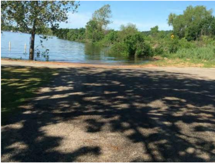
40. Bernice State Park – May 30, 2020; view southwest of north ramp. High water level recorded at 748.29 feet.
