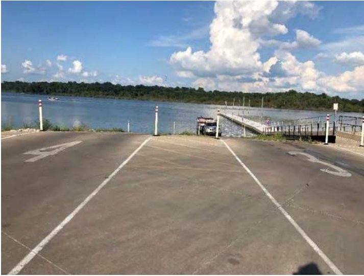
9. Wolf Creek – September 4, 2020. View northeast of boat ramps.
