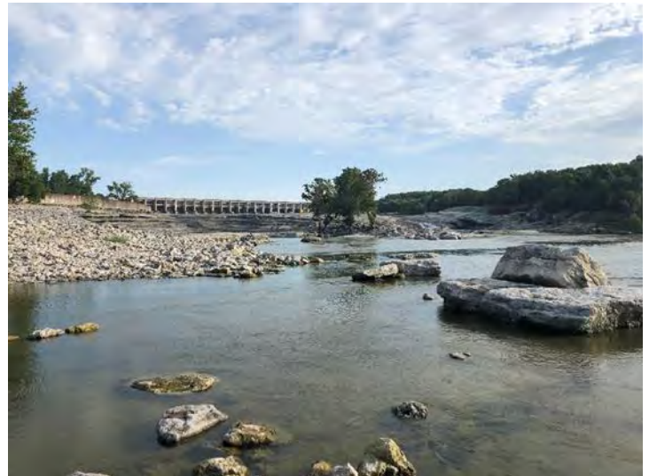
4. Channel Site – August 10, 2020. View north of Pensacola dam spillway.
