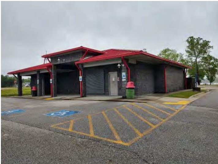
3. Wolf Creek – May 12, 2020. View north of bathroom facility with RV dump site on right side.
