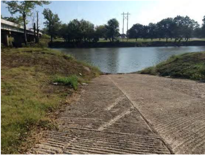
5. Riverview Park Site B – September 26, 2020; view east. Low water level recorded at 742.2 feet. (no high water mark photo from May available)
