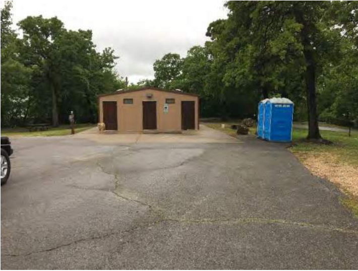
1. Cherokee State Park, Lakeside – May 12, 2020. View north of restroom/shower facility.
