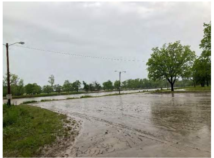
2. Riverview Park Site A – May 22, 2020. View west of parking area from top of boat ramp. Mud due to flooding.
