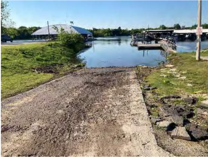
1. Willow Park – May 30, 2020. View north of boat ramp and mooring dock.
