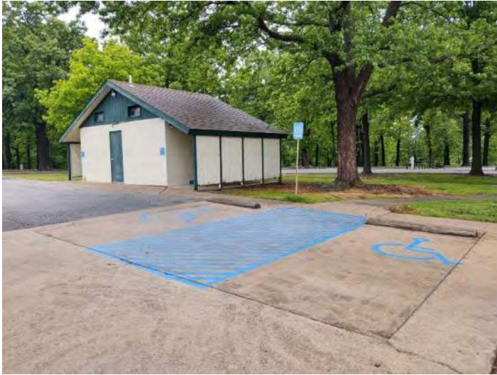
5. Honey Creek State Park – May 12, 2020. View northwest of restroom/shower facility.
