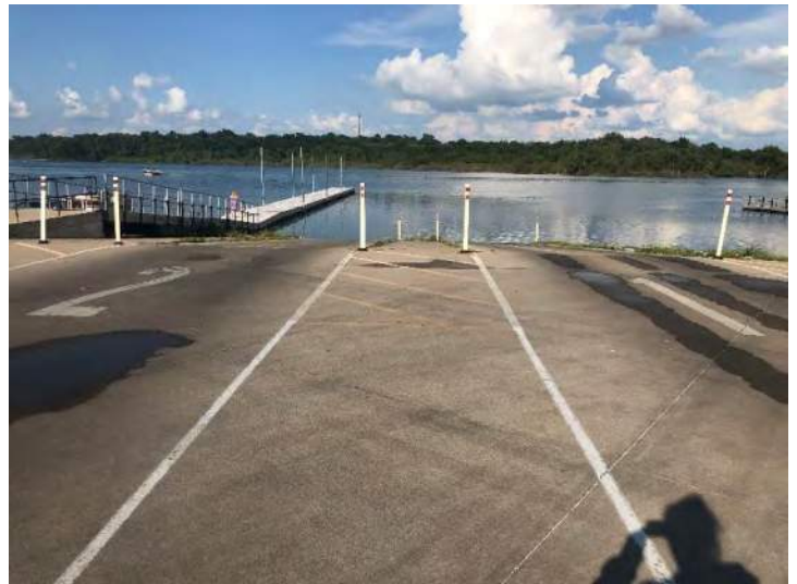
8. Wolf Creek – September 4, 2020. View northeast of boat ramps.
