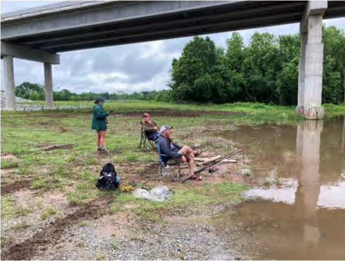
1. Spring River Public Access - May 27, 2020; view west. High water recorded on May 30, 2020 at 748.29 feet but no photo due to site flooding.
