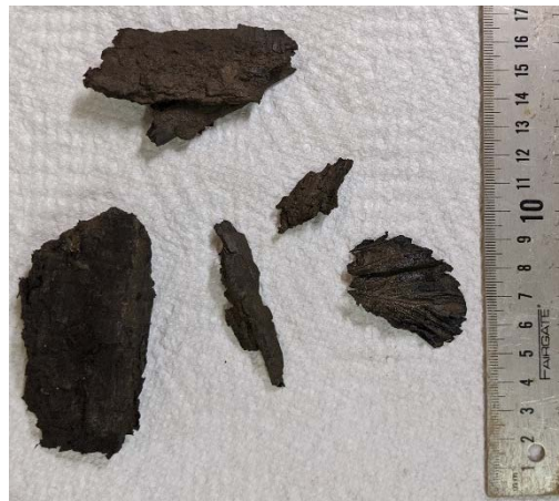
Figure 38. Wood chips found in SR-114
