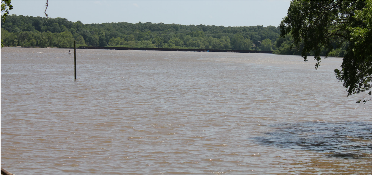
Burlington Northern Railroad Bridge and Embankment Viewed from Twin Bridges Boat Launch in May 2019
