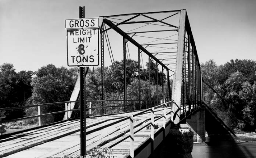
Stepps Ford Bridge (demolished 2017)
