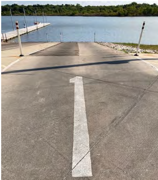
18. Wolf Creek – September 26, 2020; view northeast. Low water level recorded at 742.2 feet.
