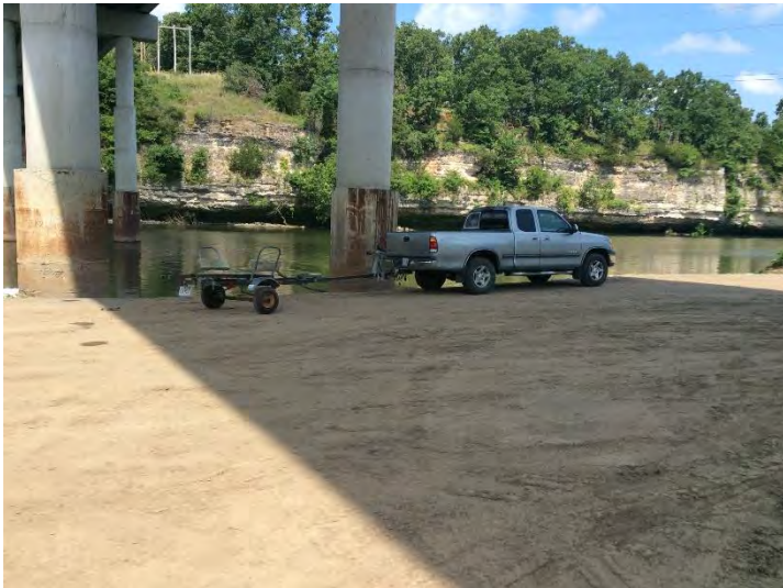
3. Spring River – July 5, 2020. View northwest from parking area.
