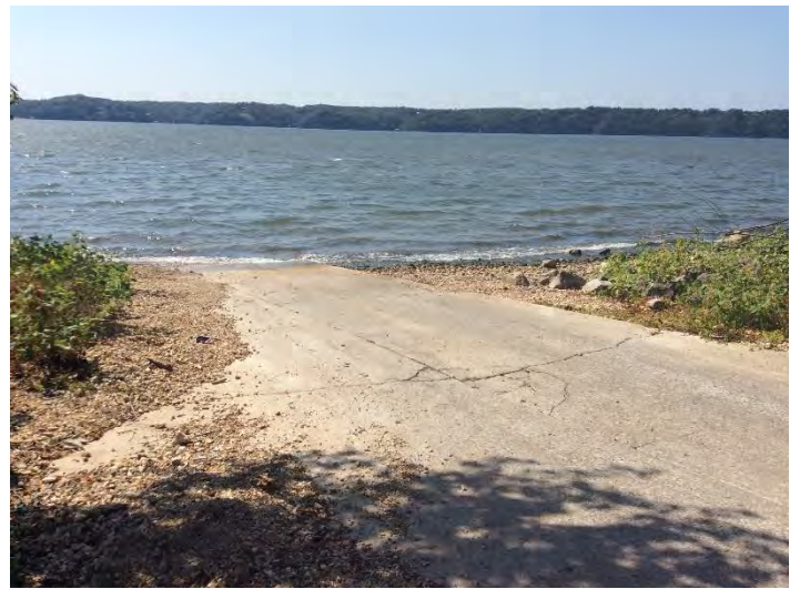
45. Monkey Island – September 26, 2020; view south. Low water level recorded at 742.2 feet.
