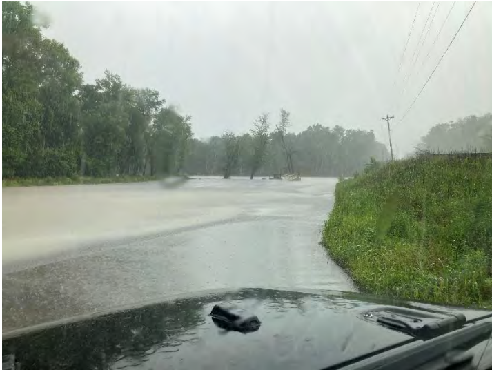
8. Connors Bridge Public Access – May 27, 2020; view south. High water level recorded on May 30, 2020 at 748.29 feet, but site was flooded/inaccessible on that date.
