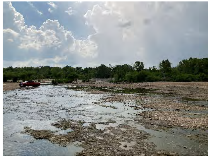
2. Channel Site – July 5, 2020. Area south of golf course.
