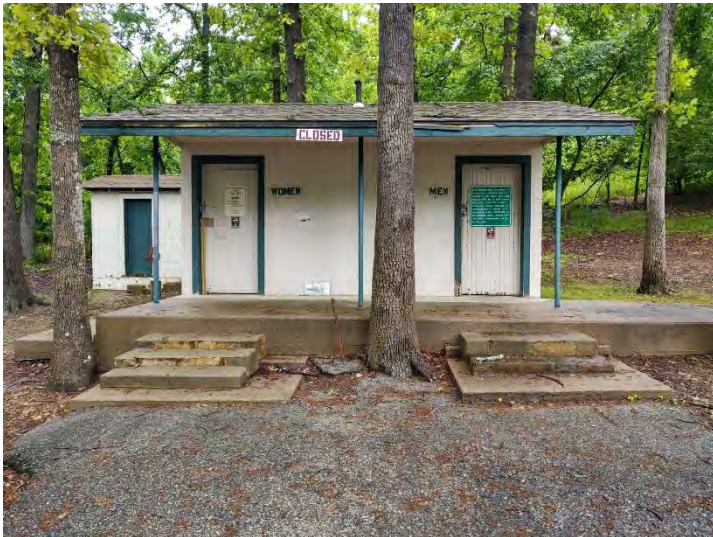
3. Honey Creek State Park – May 12, 2020. View south of restroom facility in boat trailer parking/camping area.
