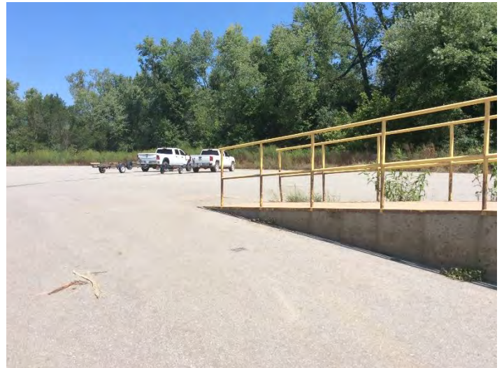
4. Connors Bridge – September 4, 2020. View southeast of parking area from boat ramp.
