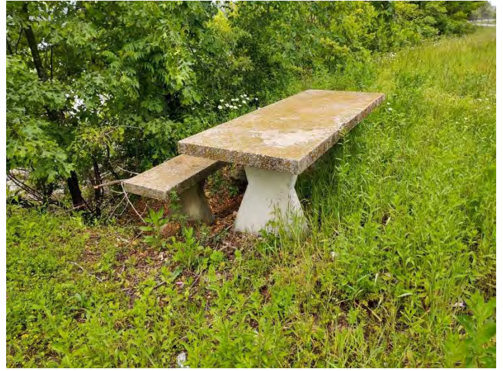
6. Council Cove – picnic table in need of replacement
