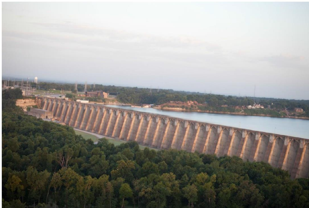
Figure 6.8-7. The multiple-arch section of the Pensacola Dam.
