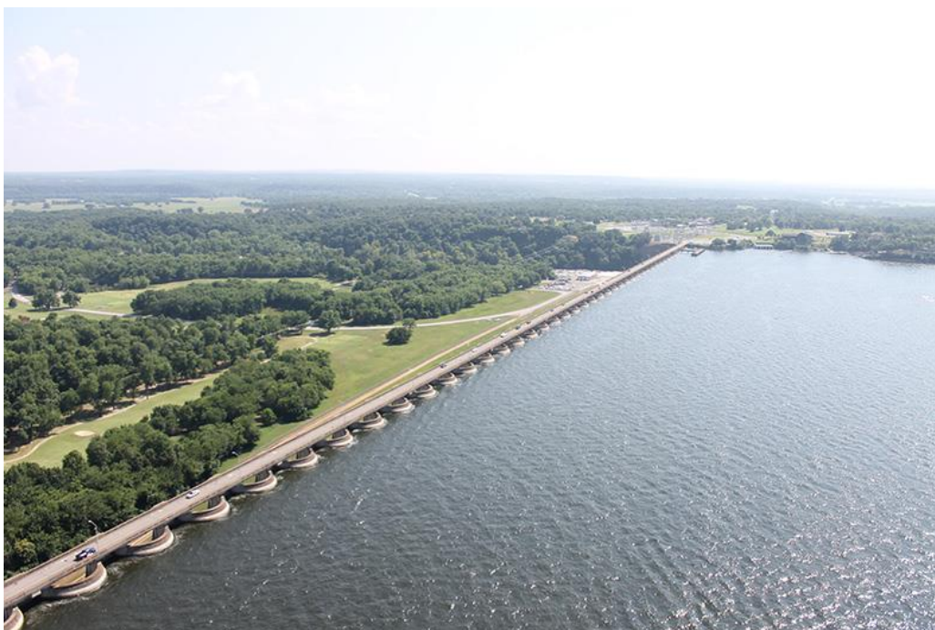
Figure 6.8-8. The highway bridge (State Highway 28) built across the length of the Pensacola Dam and the Project's east spillways, which provides two 10-foot-wide vehicle lanes and a 4-foot-wide sidewalk for pedestrians.
